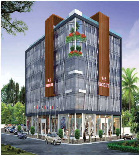
S.K.HEIGHT AT VIDYA NAGAR, HYDERABAD
