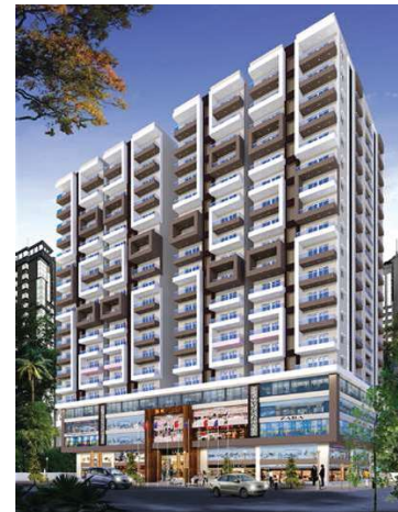
S.K.SIGNATURE SHOPPING CUM RESIDENTIAL AT GAGANPAHAD MAIN ROAD, SHAMSHABAD.
