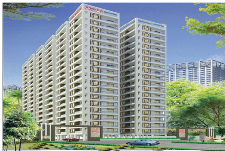
S.K.TWO AT GAGANPAHAD MAIN ROAD SHAMSHABAD
