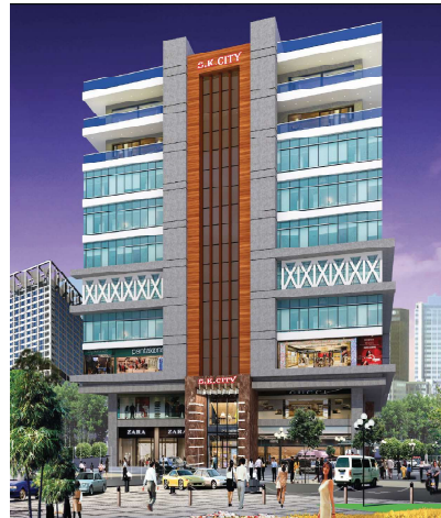
S.K.CITY SHOPPING MALL AT KANDLAKOYA, MEDCHAL
